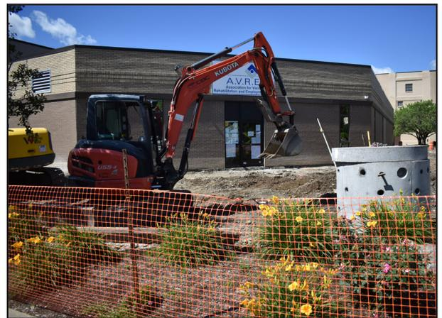
Above: An excavator removes old pavement to make way for new sidewalks and blacktop. Construction will be managed by Fahs Construction Group.
